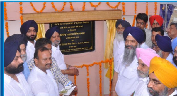
Inauguration of 220 KV Sub-station at Bassi Pathana by Hon'ble Chief Minister S. Parkash Singh Badal on 21st Sep. 2013
